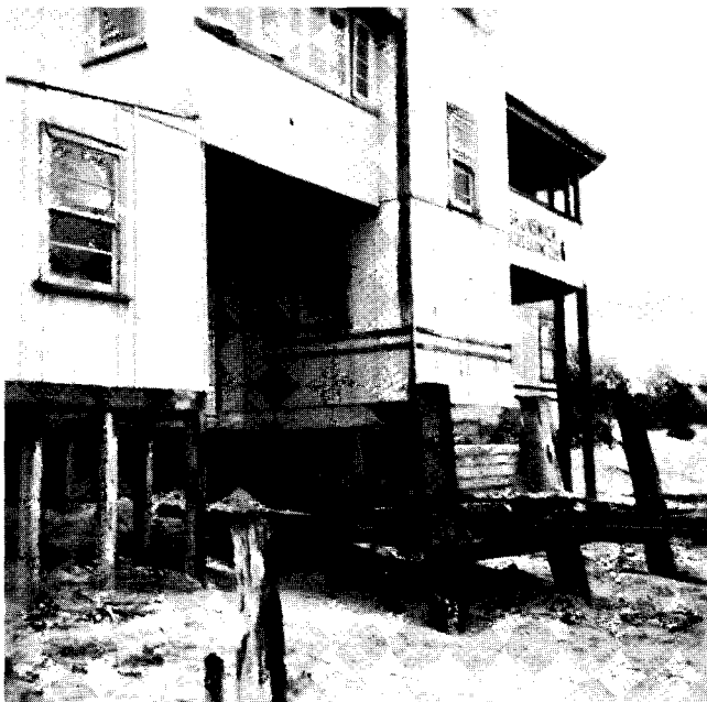
Clubhouse propped up after severe erosion. Caretaker's room on extreme left, later washed away, 1954 cyclone.
